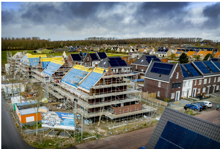
New homes being constructed in Stellendam in the Netherlands
