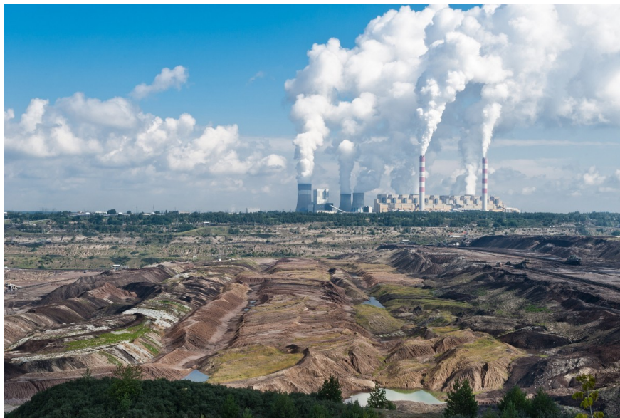
Coal power plant in Bełchatów, Poland
