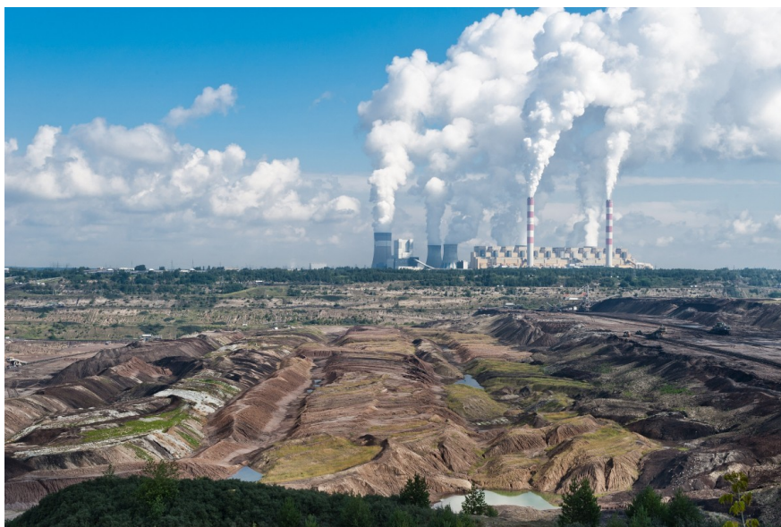
Coal power plant in Bełchatów, Poland
