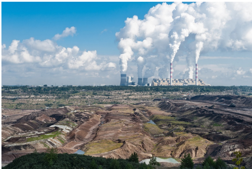
Coal power plant in Bełchatów, Poland
