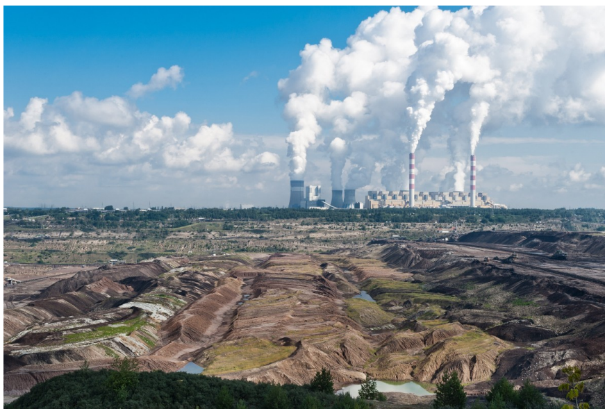
Coal power plant in Bełchatów, Poland
