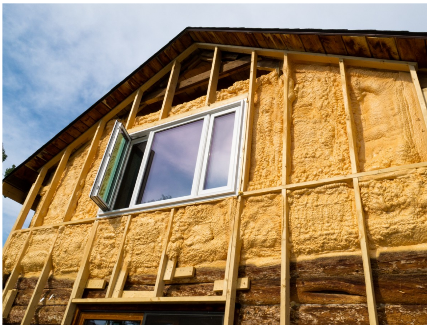
Renovation of an old home with energy efficient insulation and windows
