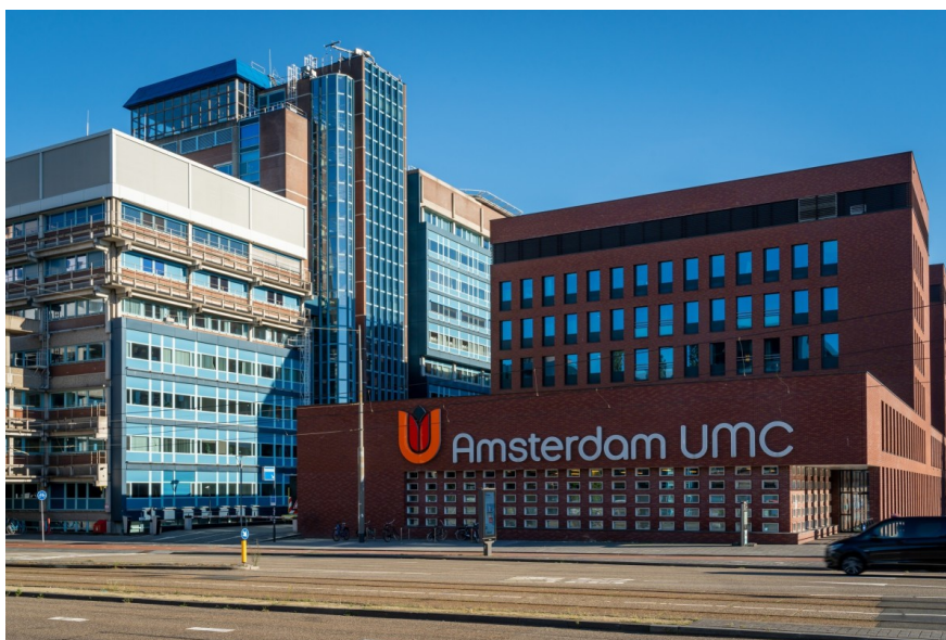
University Medical Center hospital in Amsterdam
