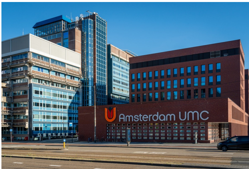
University Medical Center hospital in Amsterdam
