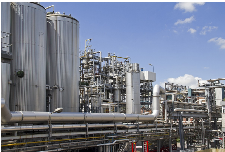
Chemical plant in Rotterdam, Netherlands
