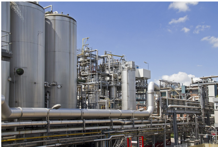
Chemical plant in Rotterdam, Netherlands
