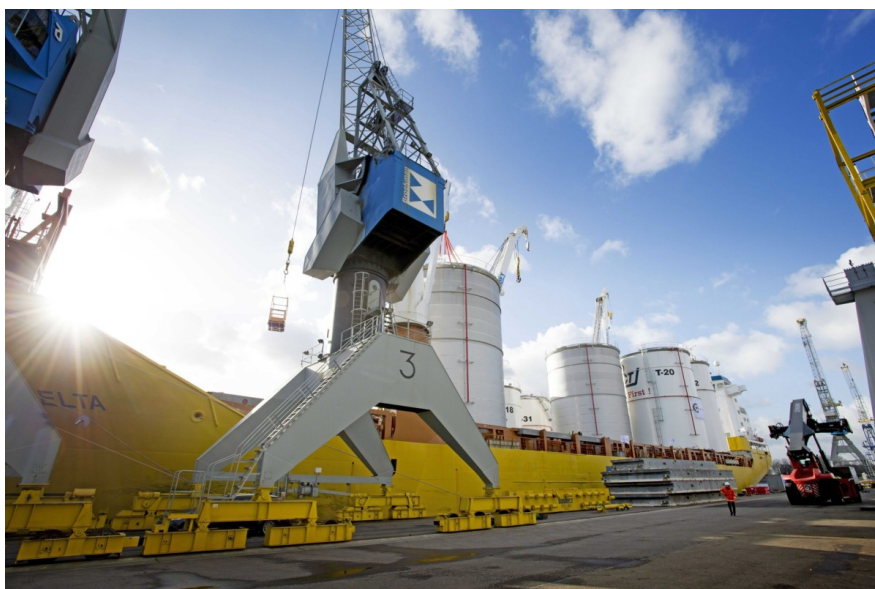
Chemical storage tanks in Rotterdam
