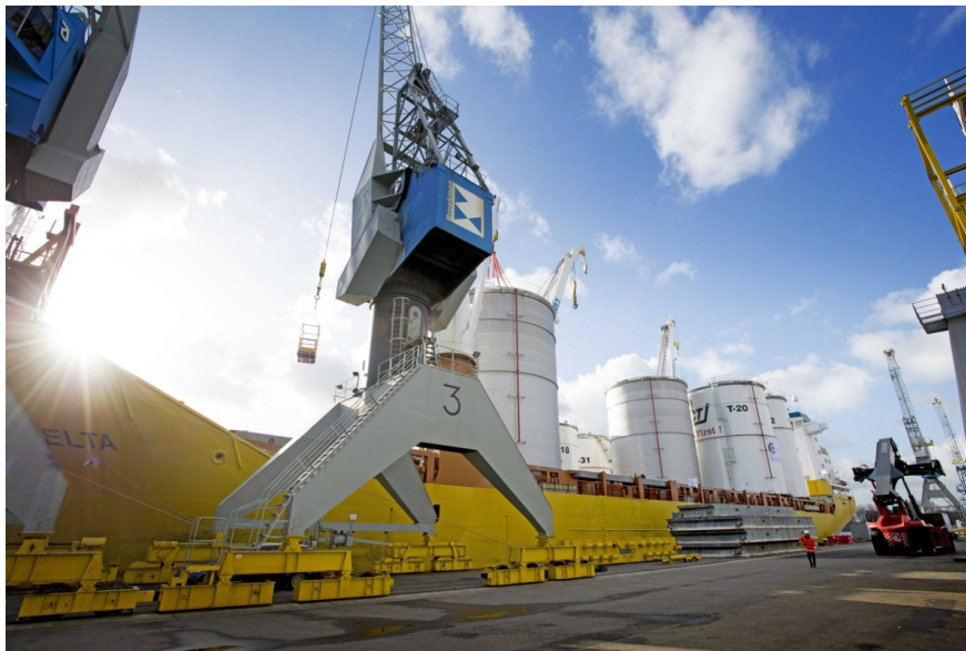
Chemical storage tanks in Rotterdam
