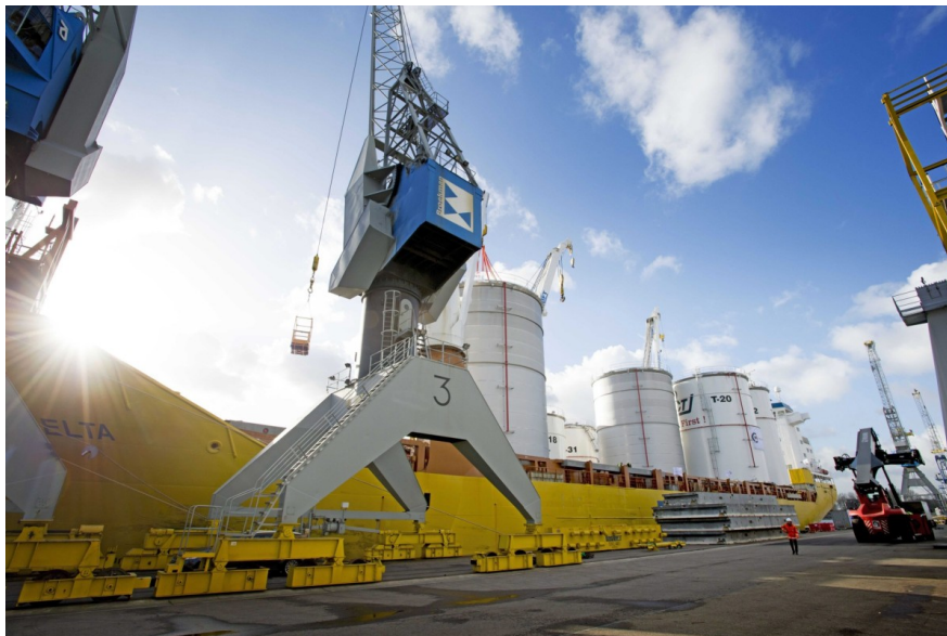
Chemical storage tanks in Rotterdam
