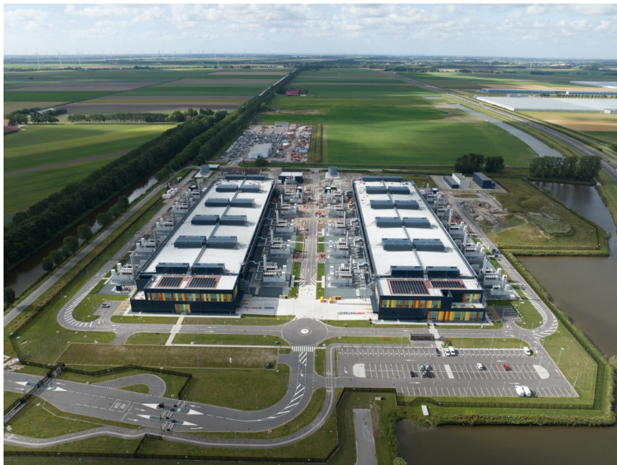
A data centre in the Netherlands
