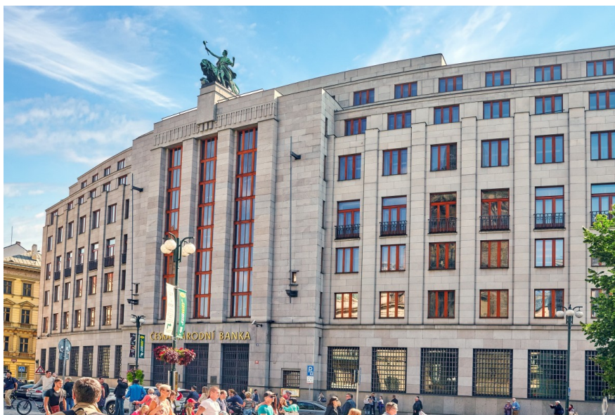
The building of the Czech National Bank in Prague
