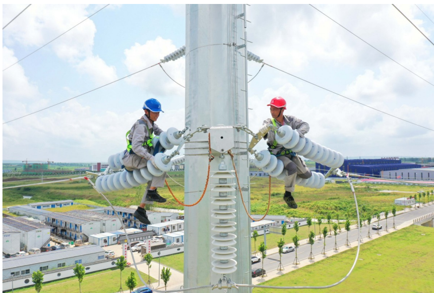
Electricity grid construction in east China, Mingguang, Anhui - 15 Sep 2021
