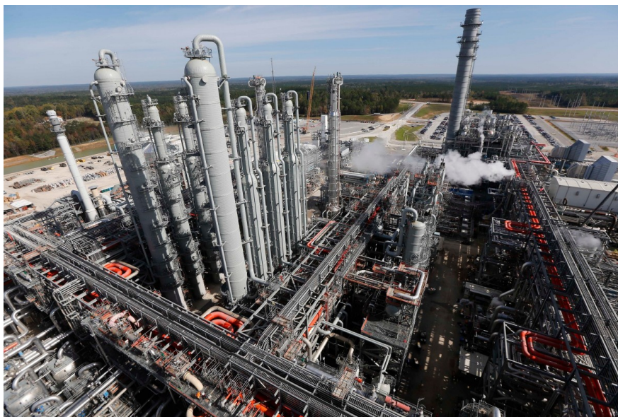
A carbon capture power plant in Mississippi in the United States
