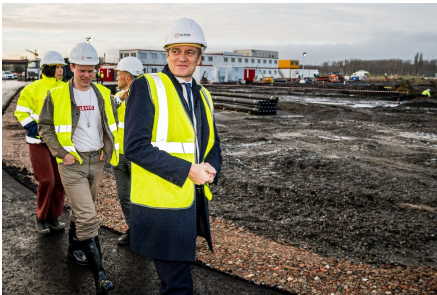
Belgium's Minister of Justice, Paul Van Tigchelt, visiting a new prison construction site in Antwerp
