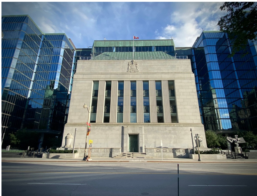
Bank of Canada building in Ottawa, Ontario
