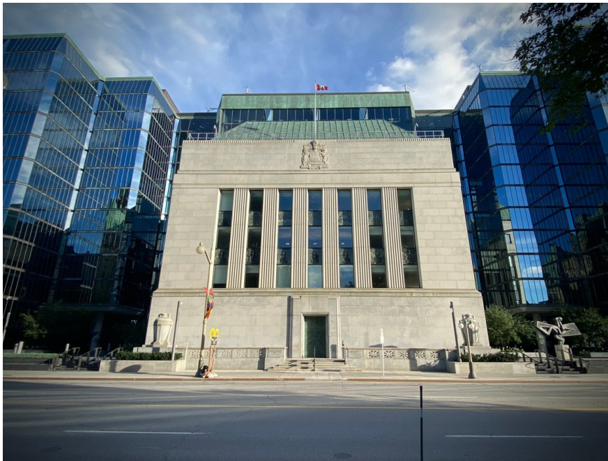
Bank of Canada building in Ottawa, Ontario
