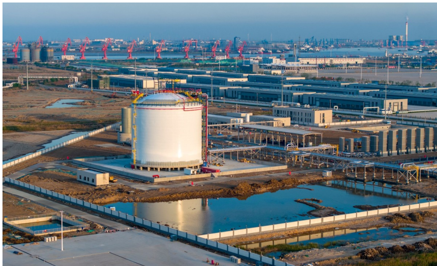
Construction is underway on the LNG storage and distribution station in China's Lianyungang City
